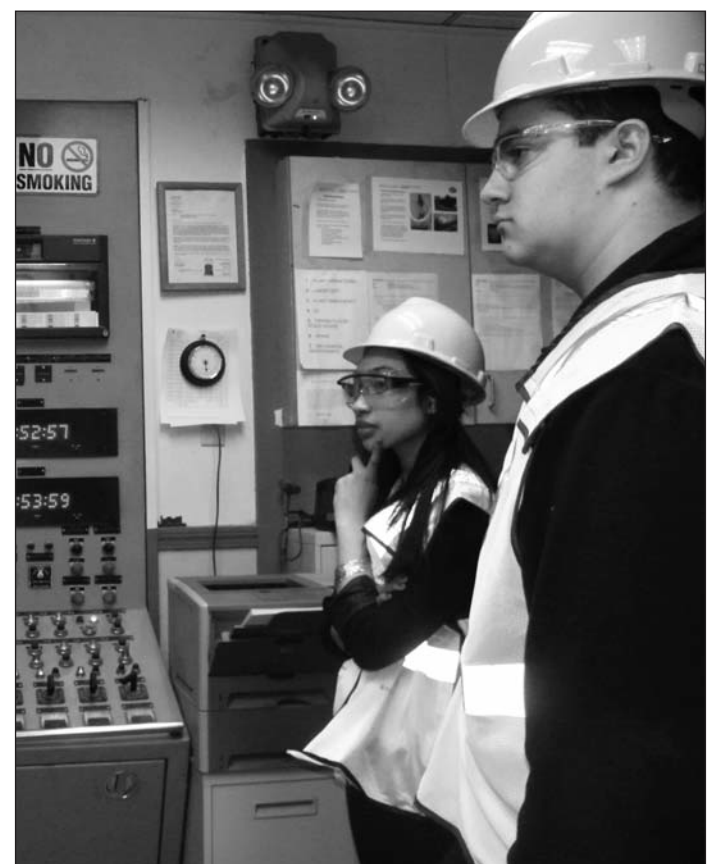
Fernandes and Downey in the control room of the plant.
