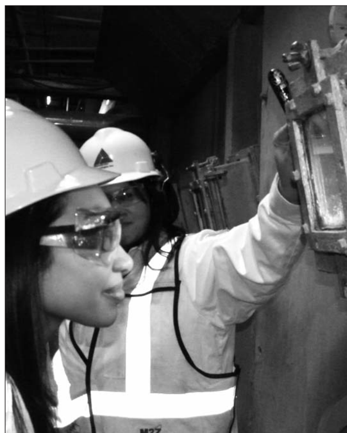
Crystal Fernandes checks out the inside of a boiler.
