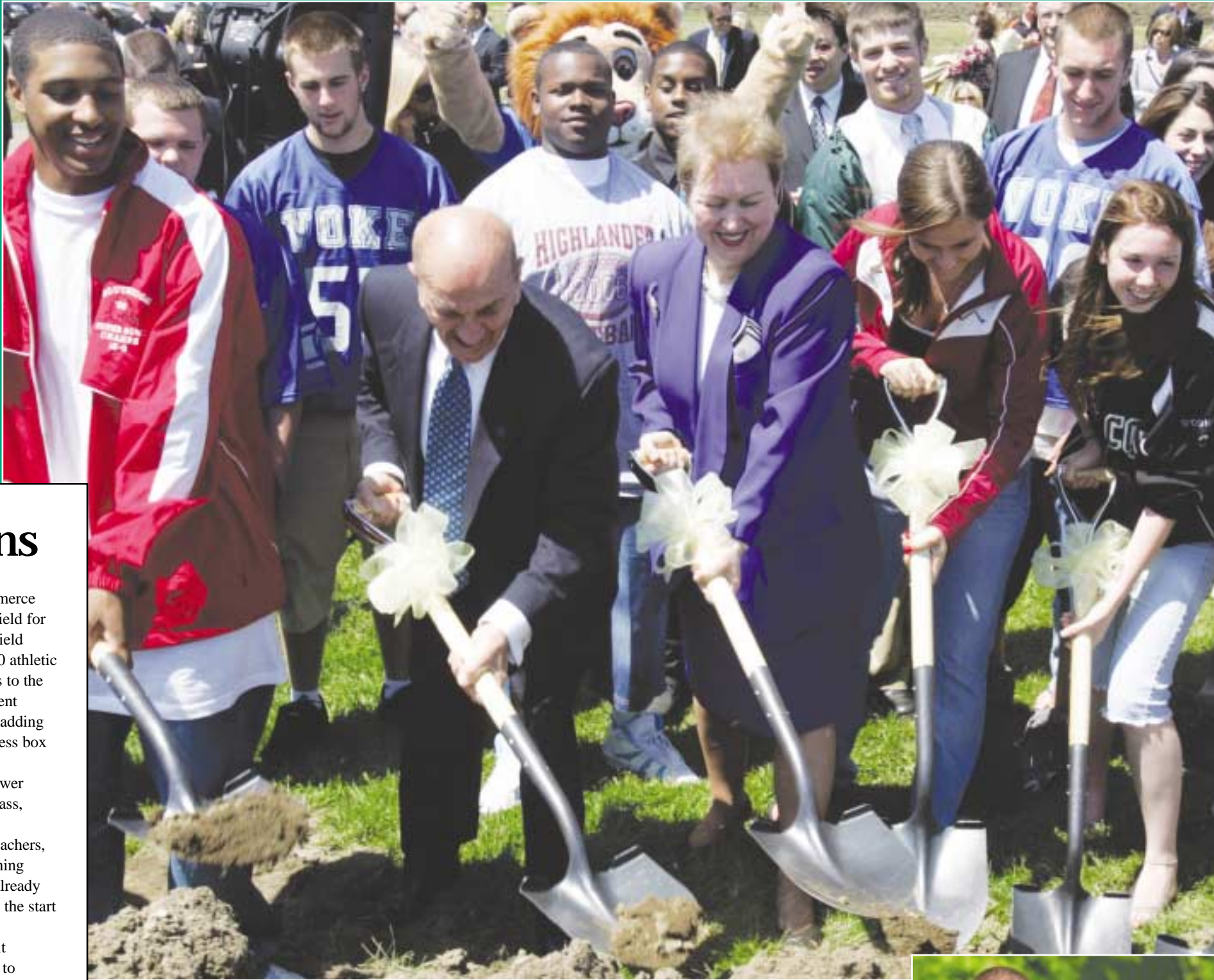
Mayor Konstantina Lukes, center, and David "Duddie" Massad of Commerce Bank, second from left, join students in the groundbreaking for the reconstruction of the field at Foley Stadium.
