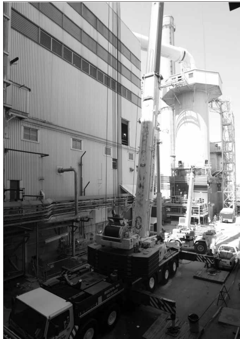
Workers perform maintenance work at Wheelabrator Saugus.
